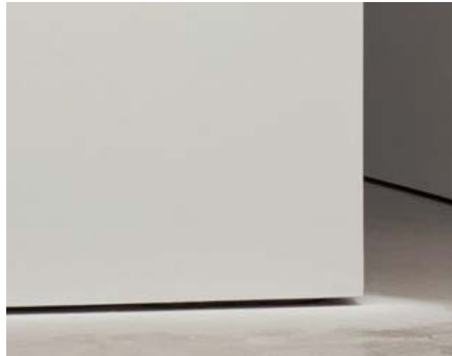
Invisible skirting board.
