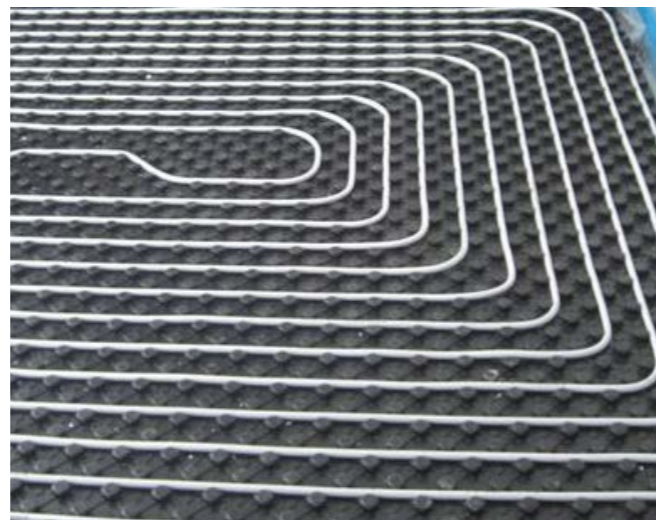
Floor heating system
